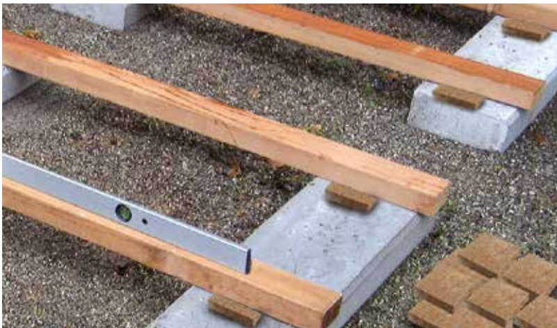
The cork-pad spacer installed in a terrace substructure.
