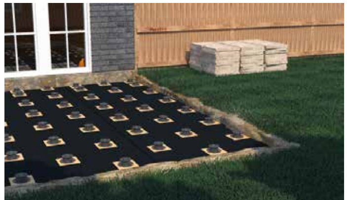
Preparation of a substructure with Profi-Line adjustable pedestals
