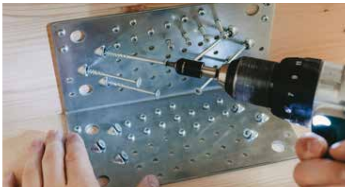
Fixing of fasteners (steel-timber connectors)
